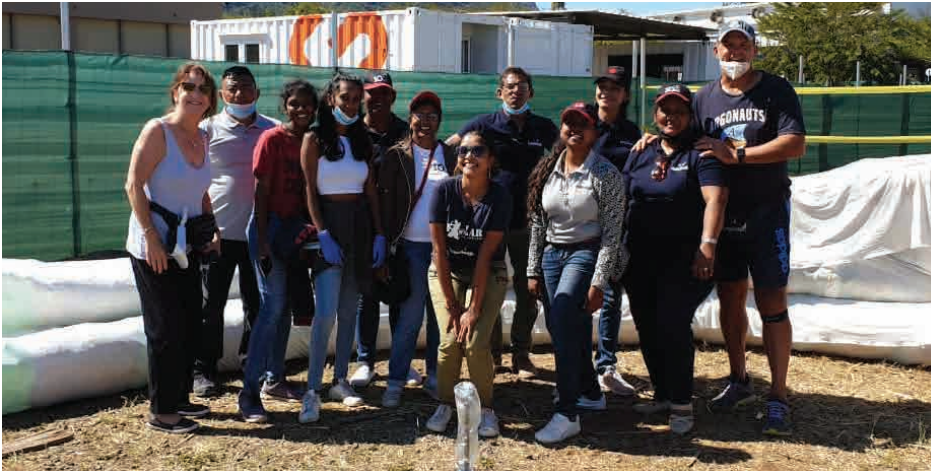
Michelle, Jan, and the team building “boom” barriers to contain the environmental disaster
